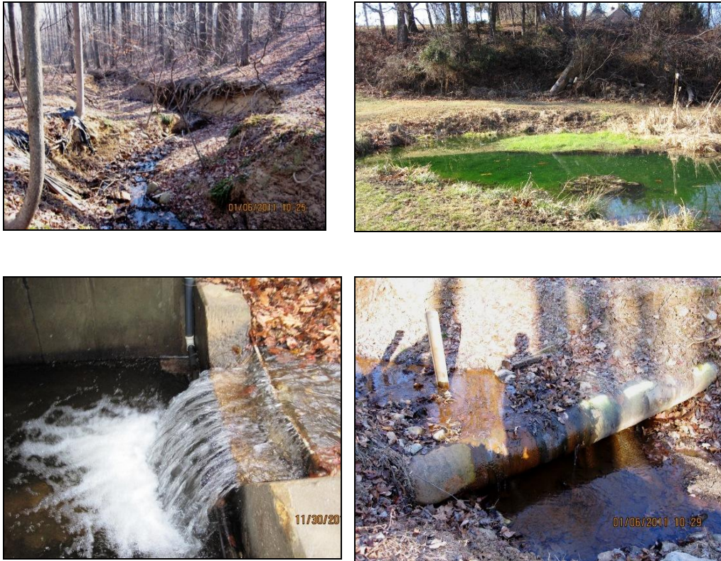
Figure 4-4: Severe problems identified in Baisman Run; Erosion site (top left), excessive algae (top right), fish migration blockage (bottom left), and exposed pipe (bottom right).
