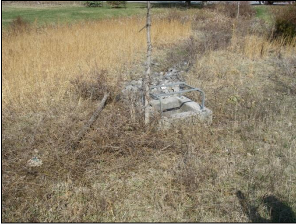
Figure 4-15: Pond #68 with concrete riser
