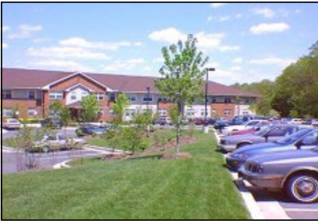
Grade changes are accommodated within parking lot medians.
