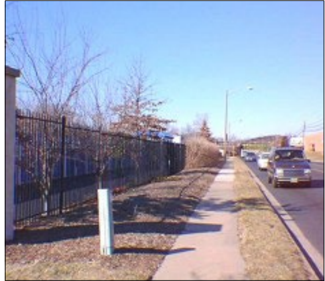
A fence with landscaping provides an effective screen for this mini-warehouse service lane.
