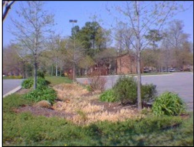
Using low impact development alternatives, stormwater management is incorporated into the parking lot medians.
