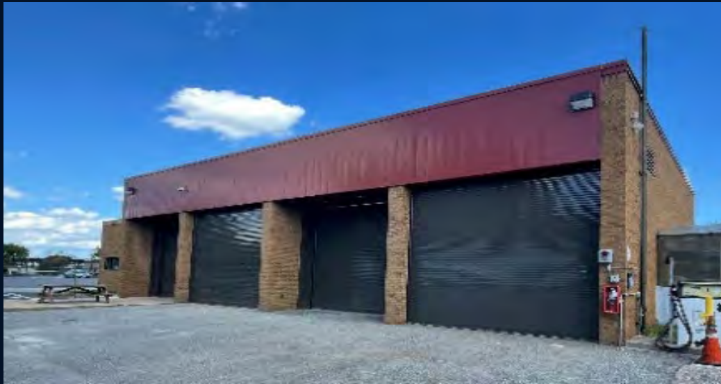
CCBC Dundalk Vehicle Maintenance Shop
