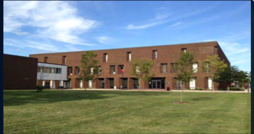
CCBC Essex Administration Building Roof Replacement
