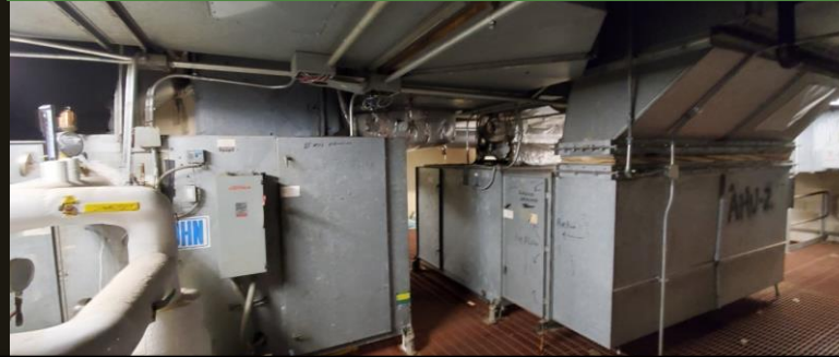
Replace and upgrade HVAC Units
