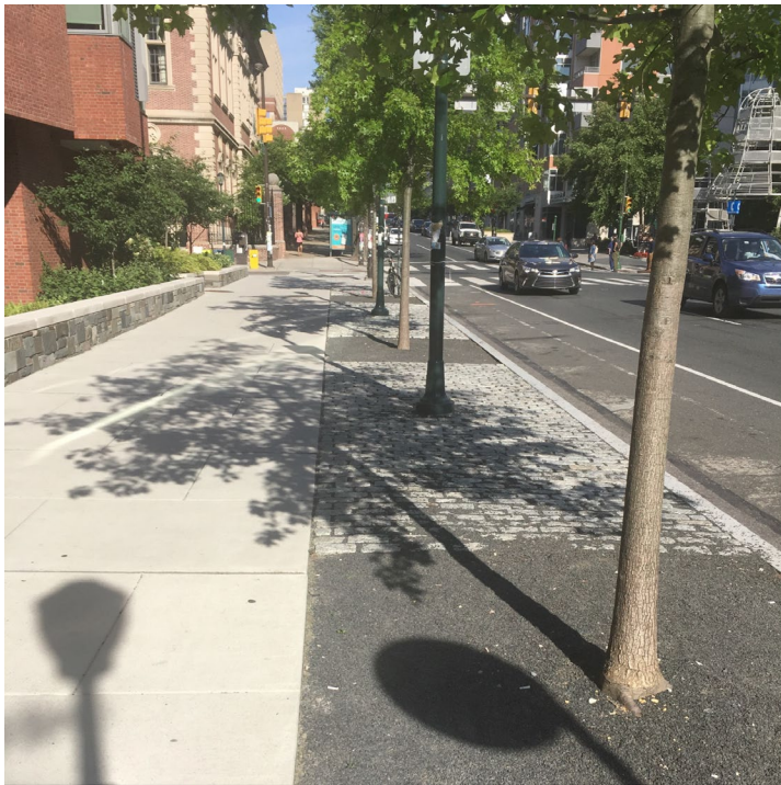
PERVIOUS PAVING USED WITH STREET TREE PLANTINGS
