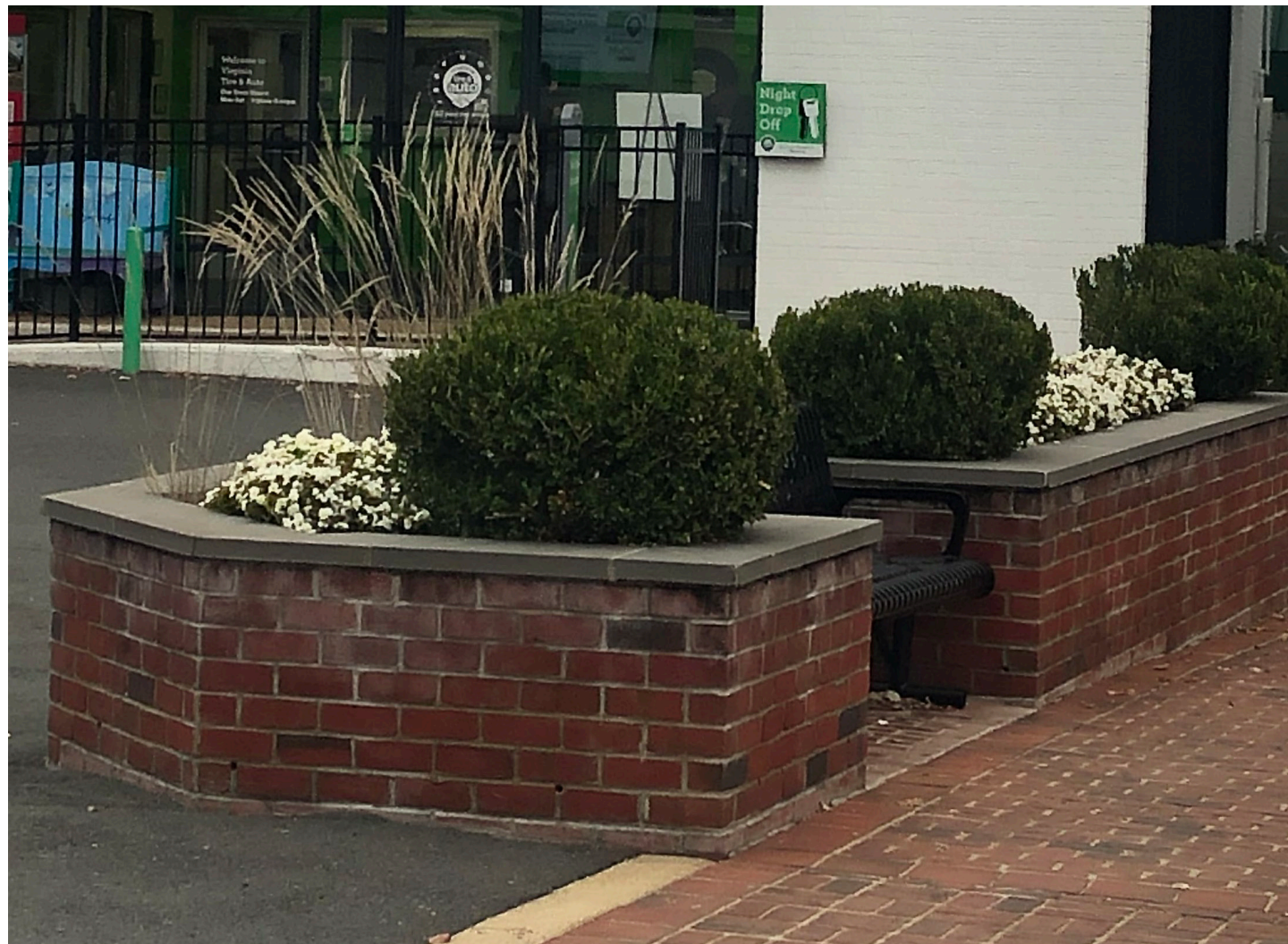
Masonry planters effectively separate the parking lot from the public sidewalk and incorporates a bench.
