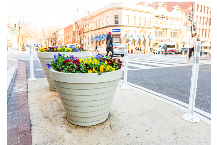
Washington, DC pedestrian improvements using painted bump outs, plastic bollards, and planters. Image Source: TerraCast
