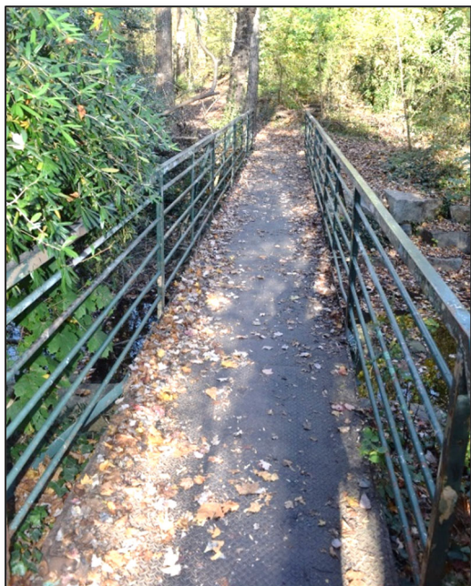
Photograph 5: Bridge 5: Greenwood Park Bridge
