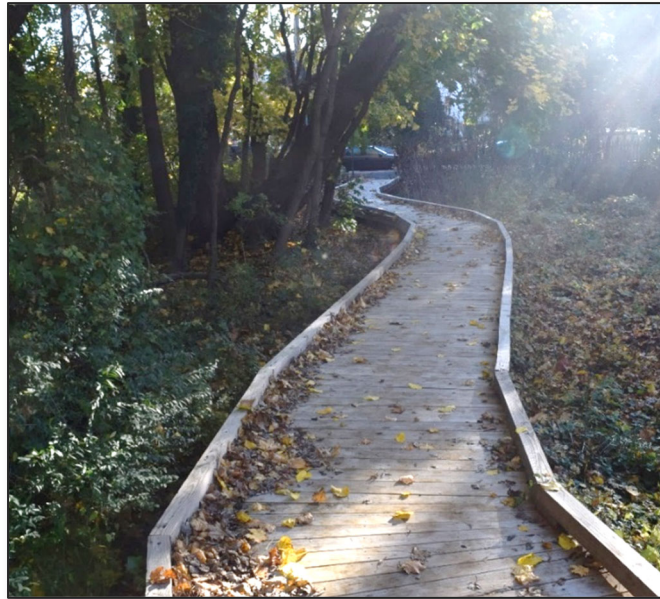
Photograph 1: Bridge 1: Radebaugh Park Boardwalk
