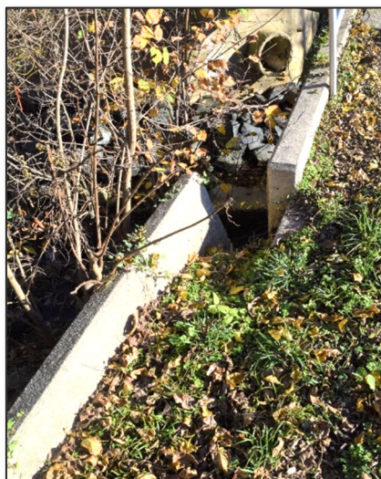
Photograph 3: Bridge 3: Northwest Wing Wall
