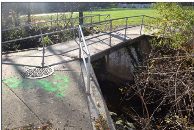
Photograph 2: Bridge 3: Towson High School North
