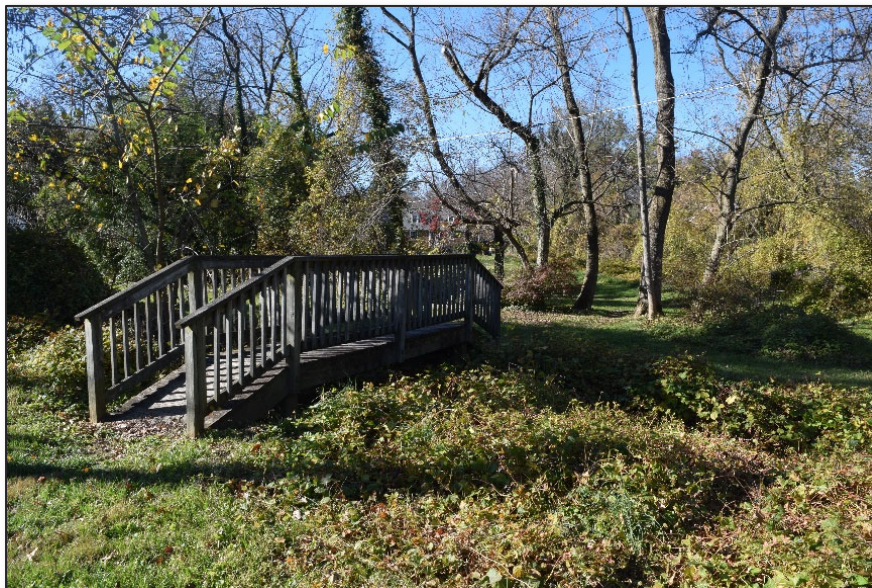
Photograph 10: Bridge 8: Footbridge near Stevenson Lane
