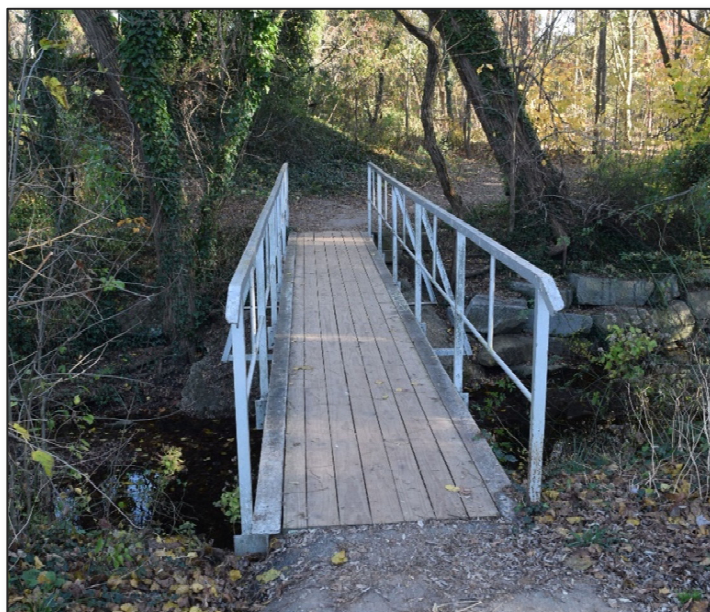
Photograph 4: Bridge 4: Towson High School South Bridge
