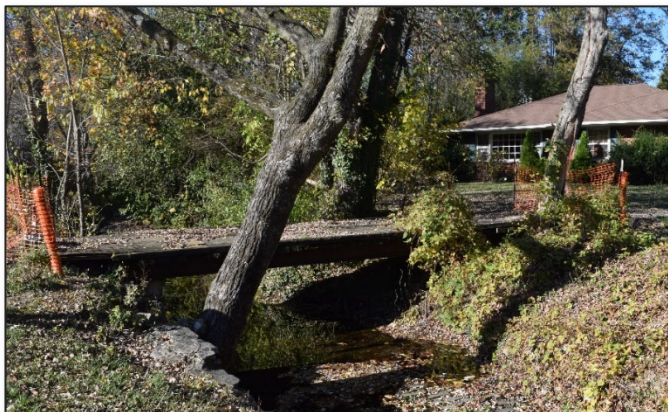
Photograph 8: Bridge 7: Worthington Road
