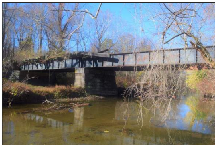
Image 14: Existing Bridge over Western Run
