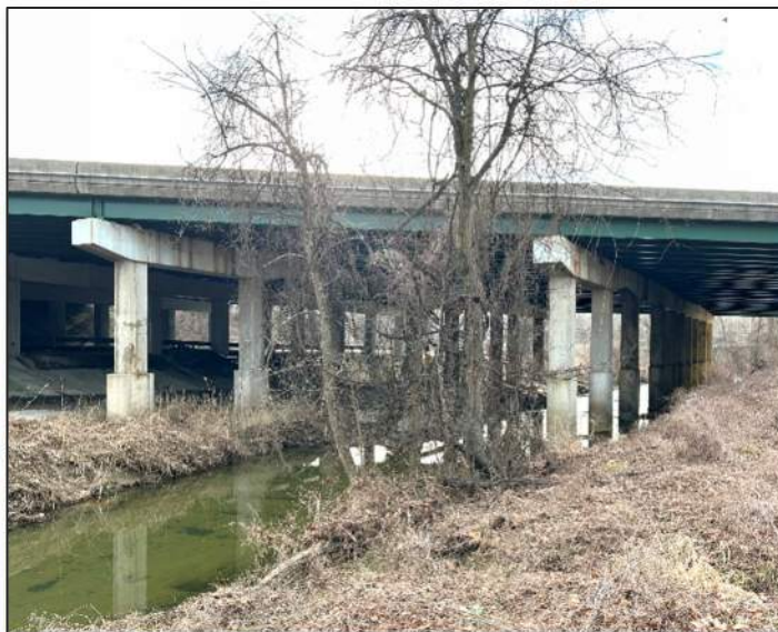
Image 9: I-695 overpass of JFX and Jones Falls
