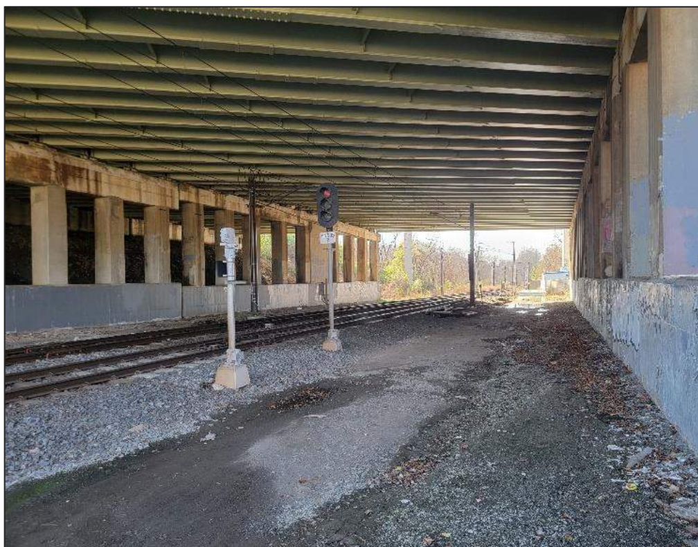
Image 20: I-695 Overpass of the Light Rail near Seminary Park
