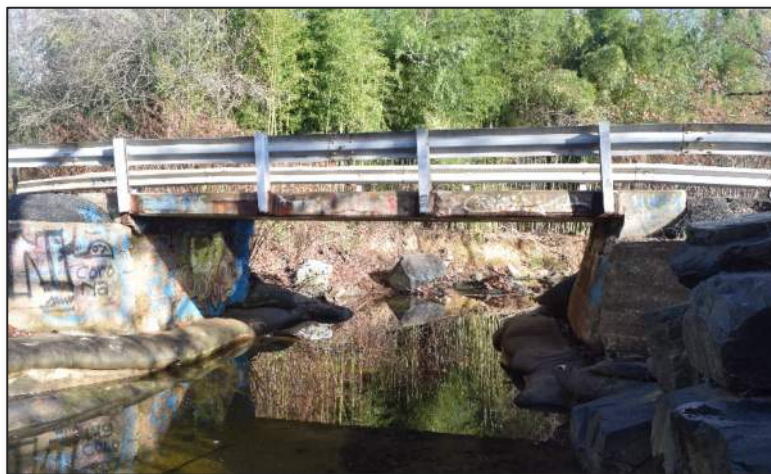
Figure 15: Existing bridge over Stemmers Run
