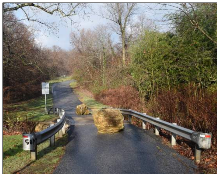
Figure 4: Existing bridge over Stemmers Run
