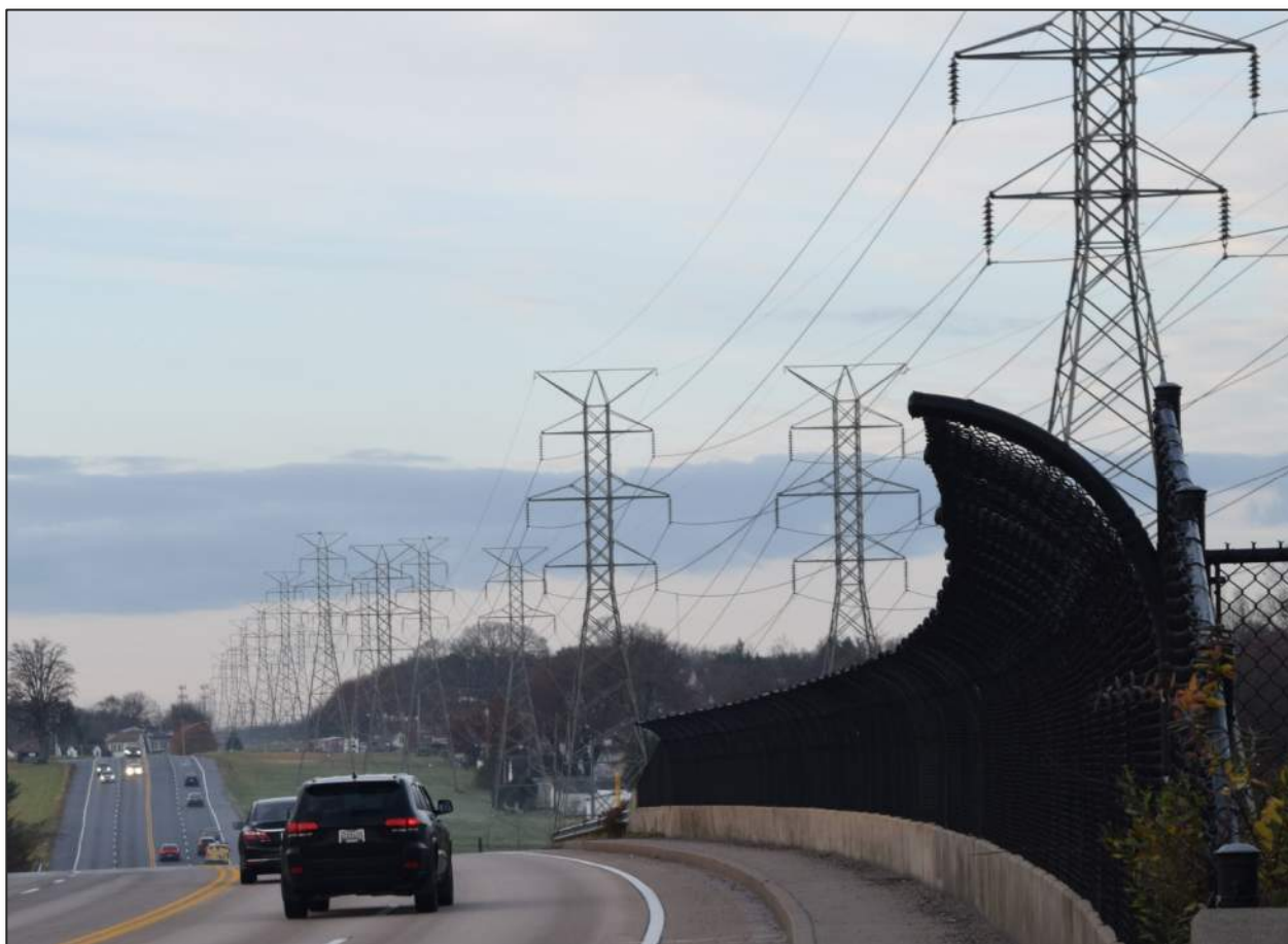
Figure 3: Utility corridor along Lillian Holt Drive
